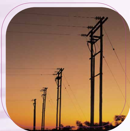
Expansion of electrical distribution infrastructure in rural areas.
